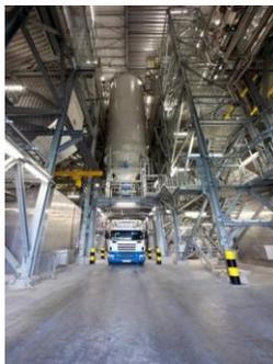
The resultant residue left on the filter bags is termed Air Pollution Control residue (APCr) and this is collected in 3 silos. APCr accounts for approximately 3-4% of the facility's waste throughput and in 2017 the facility recycled approx. 50% of the APCr produced at site. The remainder of the APCr was sent for disposal at a licensed hazardous waste site.
