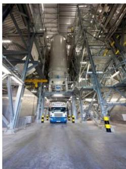
The resultant residue left on the filter bags is termed Air Pollution Control residue (APCr) and this is collected in 3 silos. APCr accounts for approximately 3-4% of the facility's waste throughput and in 2015 the facility recycled approx. 50% of the APCr produced at site. The remainder of the APCr was sent for disposal at a licensed hazardous waste site.
