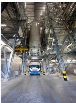
The resultant residue left on the filter bags is termed Air Pollution Control residue (APCr) and this is collected in 3 silos. APCr accounts for approximately 3-4% of the facility's waste throughput and at present and is sent for disposal at a licensed hazardous waste site. In 2014, methods for recycling APCr were trialled and, after proving to be successful, the facility now recycles 40-45% of the APCr produced at site.
